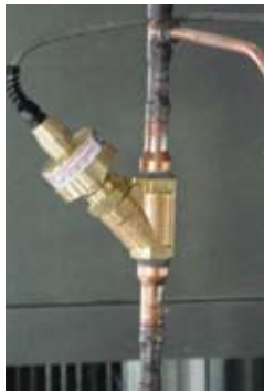
Modulating Control Valve
