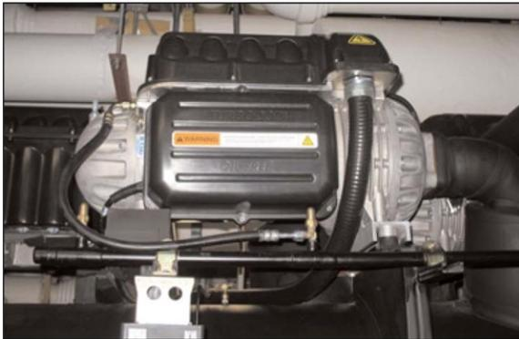
The Danfoss Turbocor Compressor (5 on each SMARTD Chiller) features Oil-free Compressor Technology
