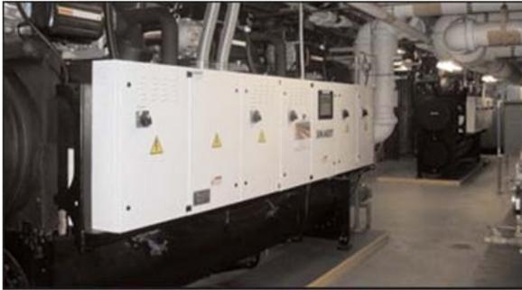
450-ton SMARTD Chiller featuring 5 Danfoss Turbocor Compressors
