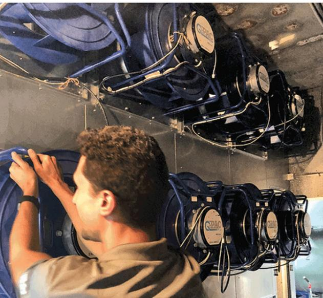
The maintenance manager was seeking a fan system solution that would not require special cranes, rigging nor demolition of the existing building. He hoped to replace the fan then install new filtration and UV lights while keeping the existing shell of the AHU.
